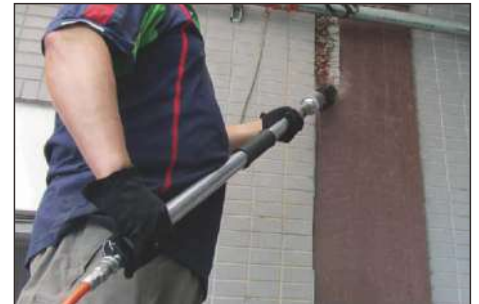
Corrosion removal for inaccessible area
